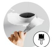
trimless installation in plasterboard
