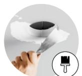
trimless installation in plasterboard
