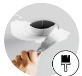
trimless installation in plasterboard
